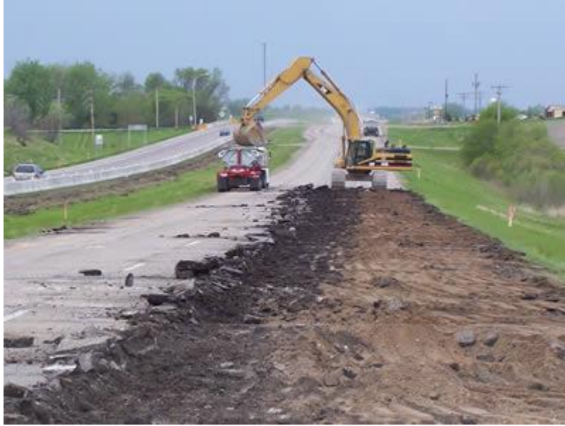
Figure 4.8: Pavement Reconstruction
