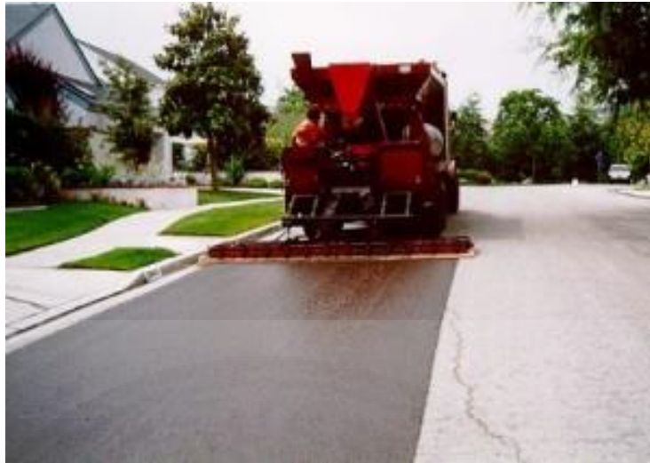
Figure 4.6: Slurry Seal
