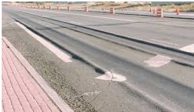
Figure 4.3: Rutting Pavement
