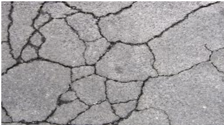
Figure 4.4: Cracked Pavement (Internet source: wallpaperweb.org )
