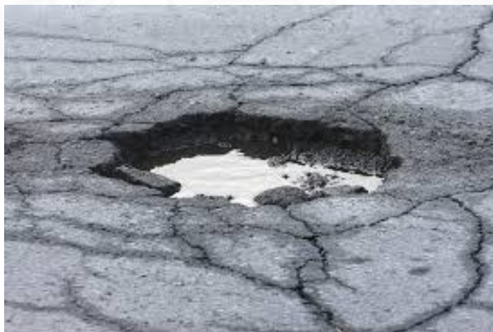
Figure 4.1: Pothole
