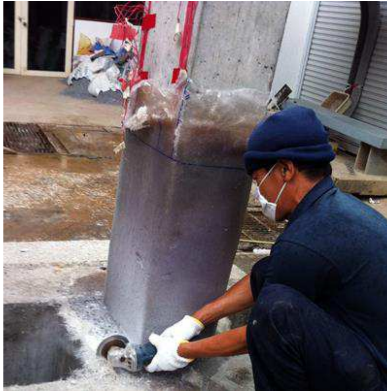
Figure 12-6: SFRP cutting process
