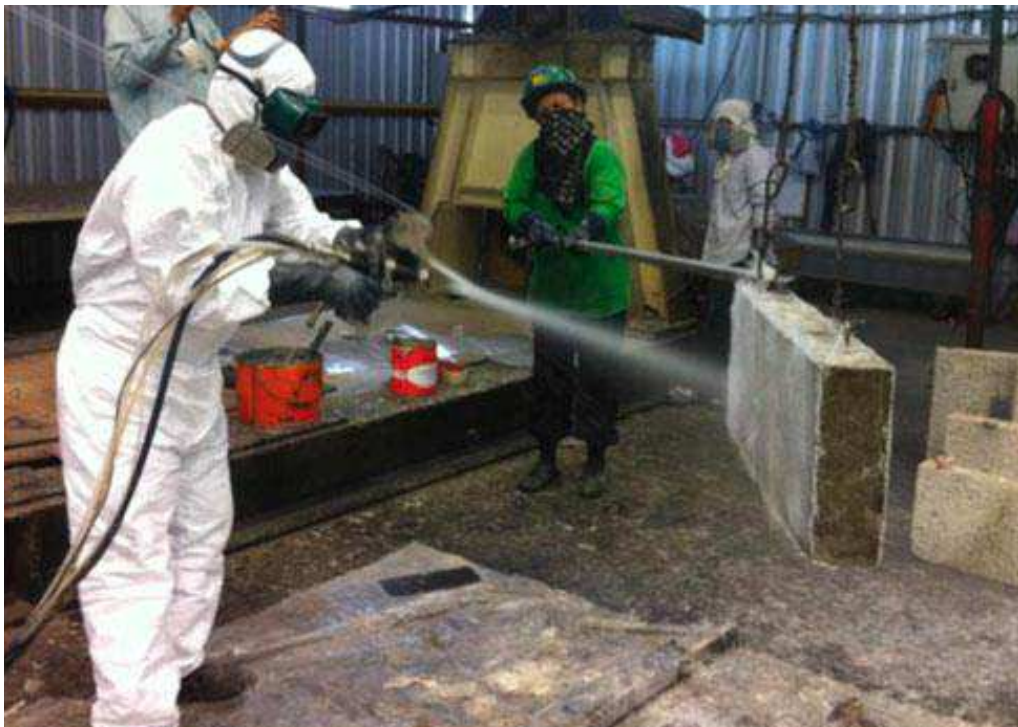
Figure 8-4: Spraying process of FRP
