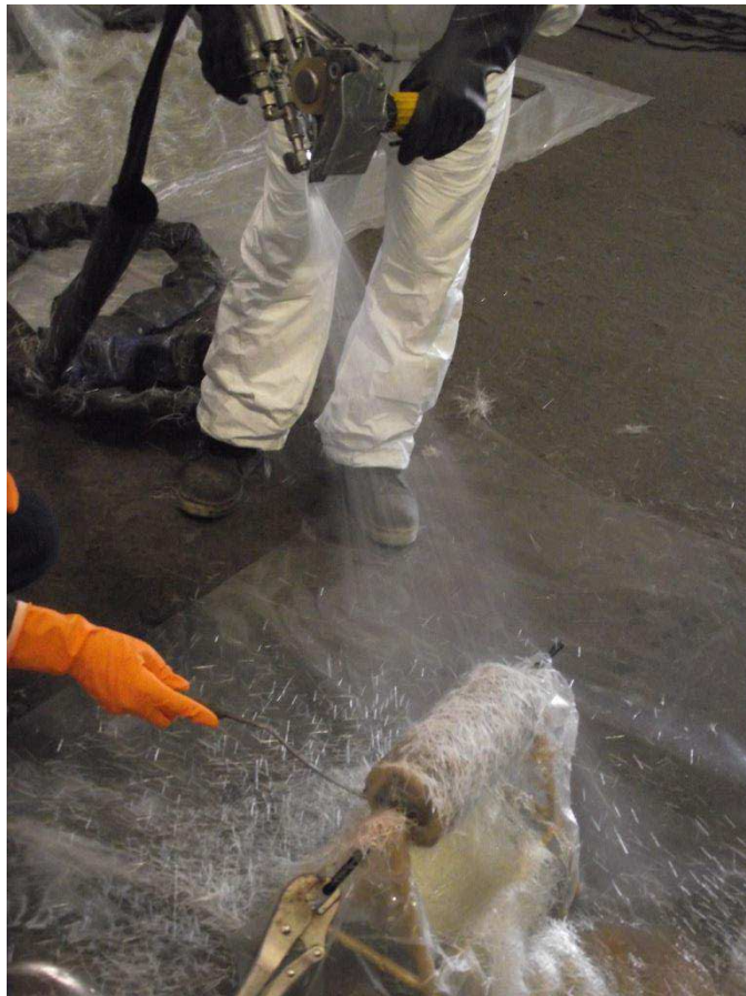
Figure 6-5: SFRP application process
