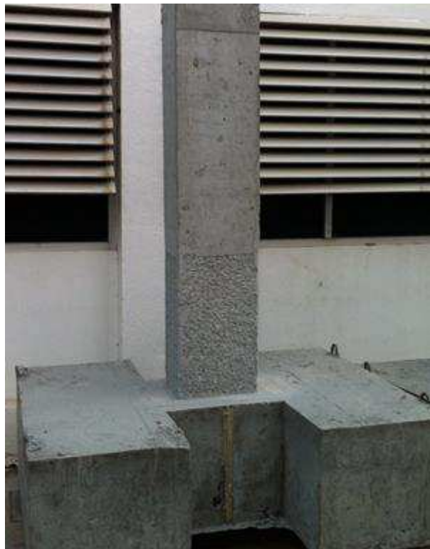
Figure 12-3: Roughened concrete surface of column
