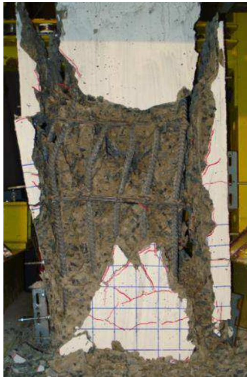
Figure 12-23: Failure mode of column SD-CON at 3.5% lateral drift
