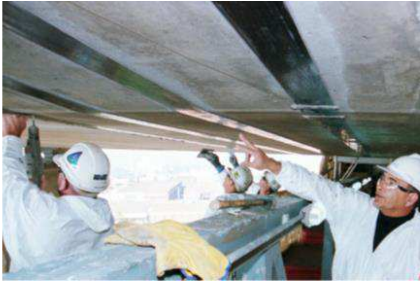
Figure 1-3: Application of Carbon FRP to the box girder [14]
