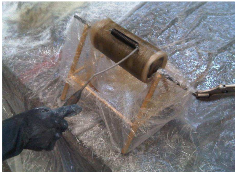
Figure 4-7: A ribbed aluminum roller is used to obtain uniform thickness of SFRP on cylinders
