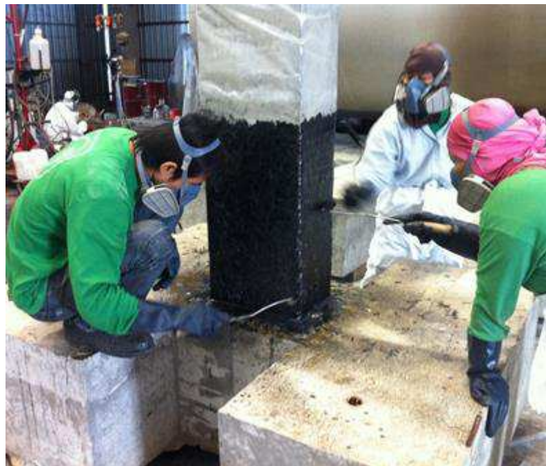
Figure 12-5: Surface preparation using ribbed aluminum roller
