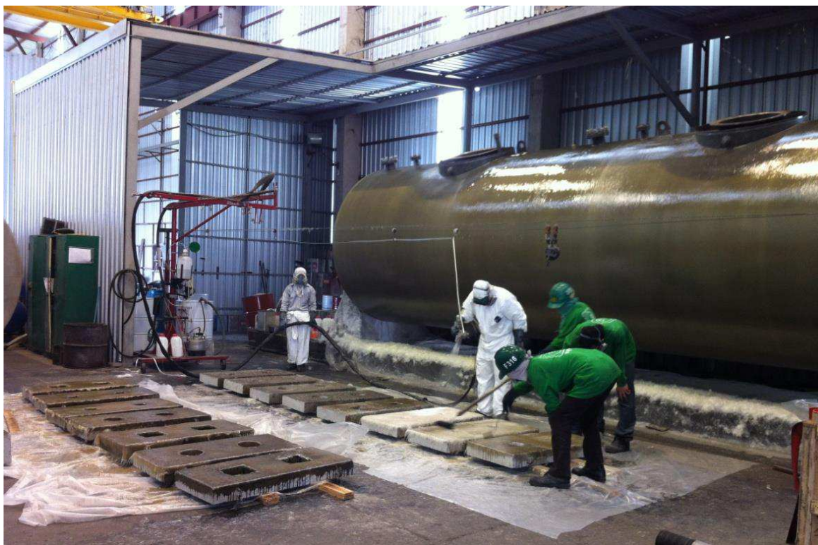
Figure 9-6: SFRP strengthening process of RC deep beams with openings
