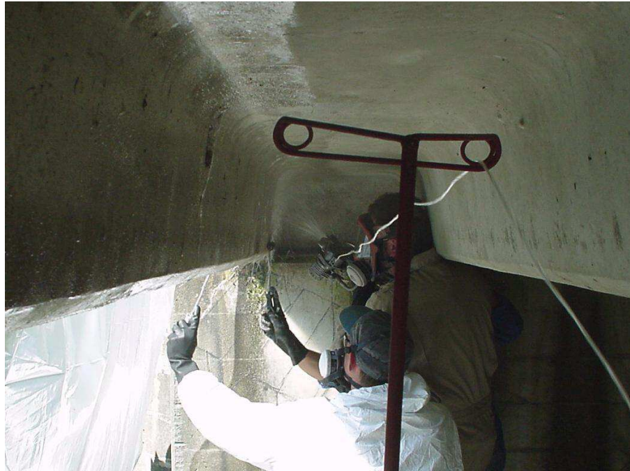
Figure 2-5: Application of SFRP on girders
