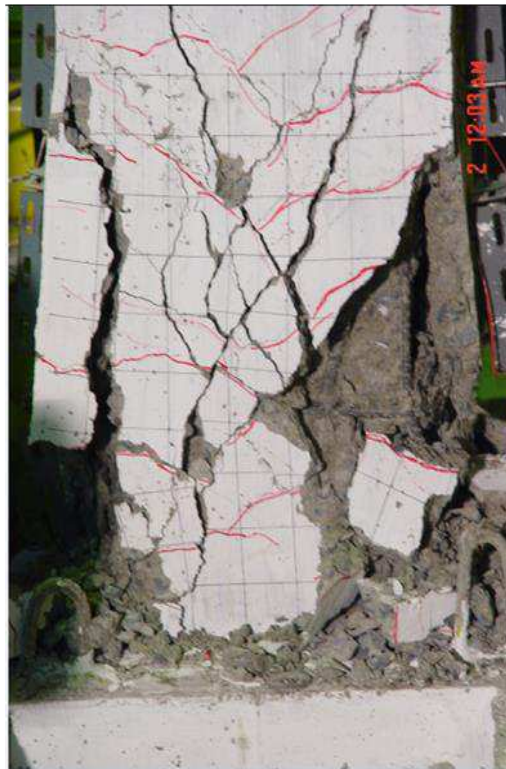
Figure 12-25: Failure mode of column FSD-CON at 4% lateral drift
