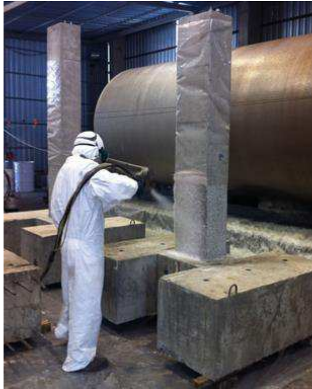
Figure 12-4: SFRP application process
