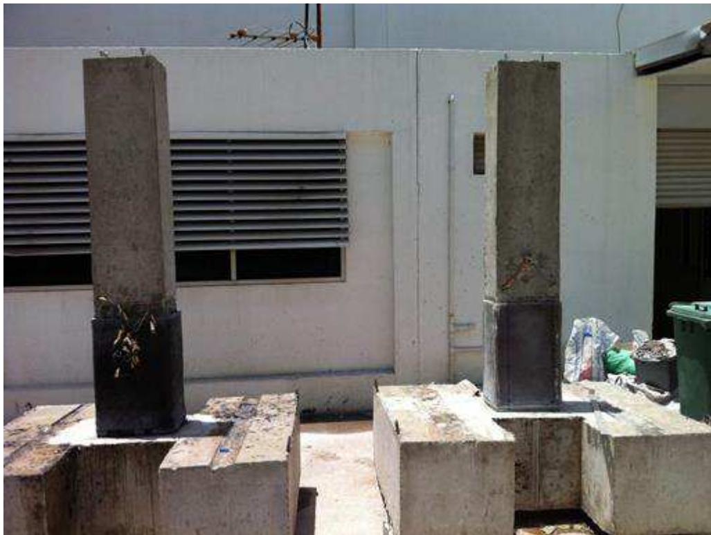
Figure 12-7: SFRP strengthened RC Columns
