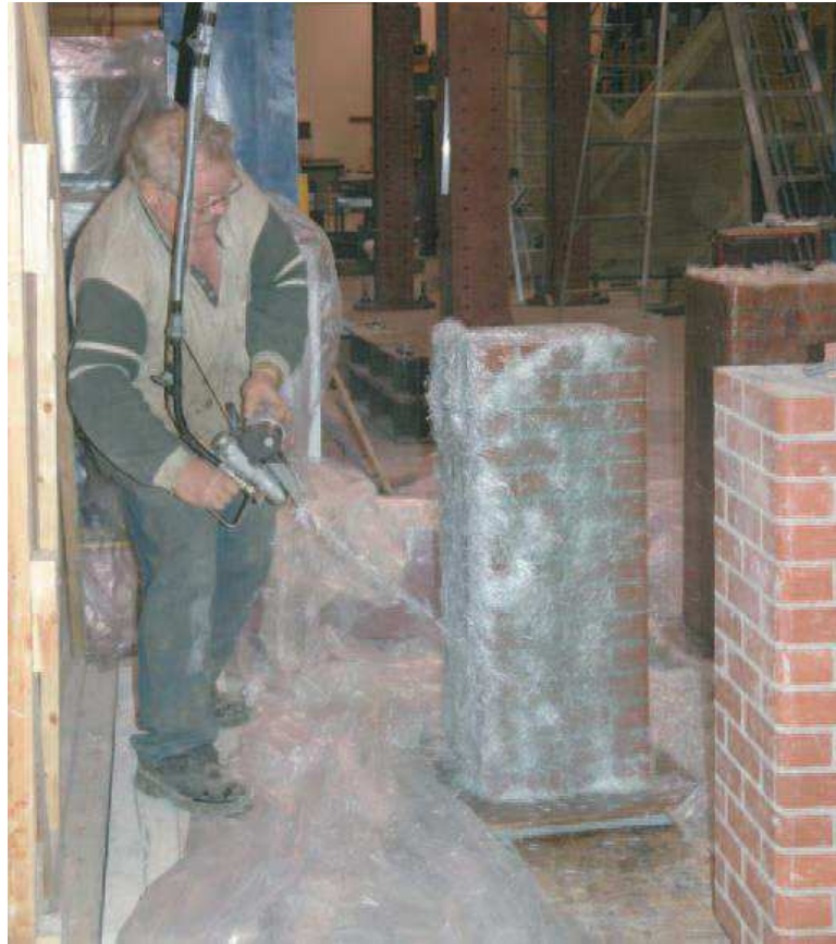
Figure 2-11: Glass fiber reinforced polymer spraying process
