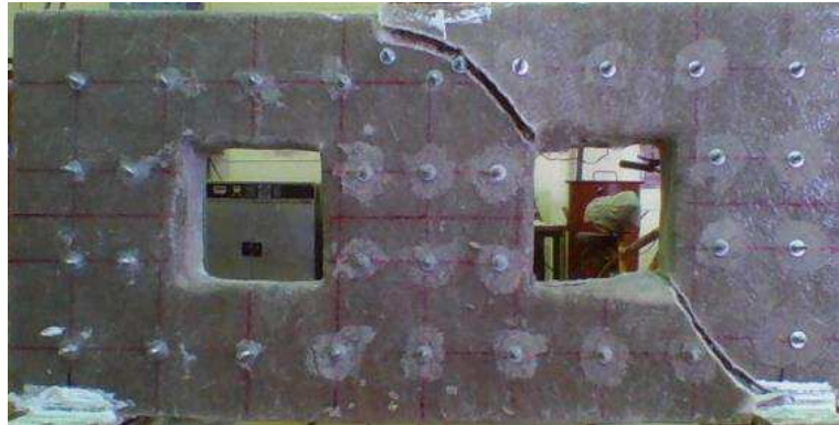
Figure 9-16: Typical failure mode of SFRP strengthened beam specimen of group A
