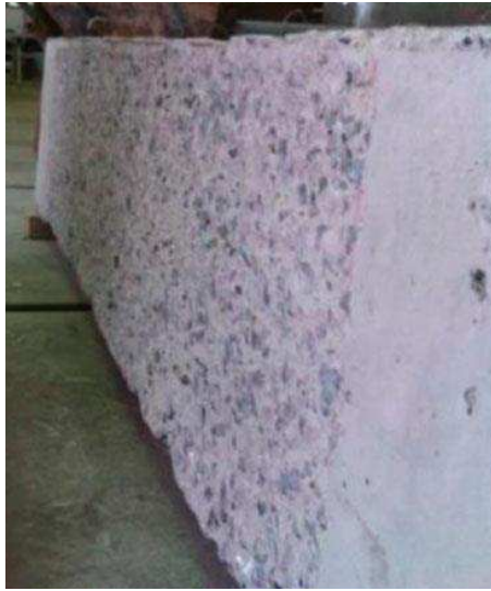
Figure 8-3: Roughened Concrete surface of beam
