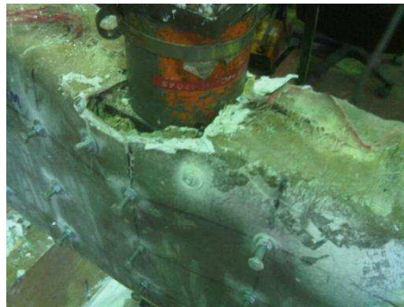
Figure 8-21: Typical concrete crushing failure under loading region
