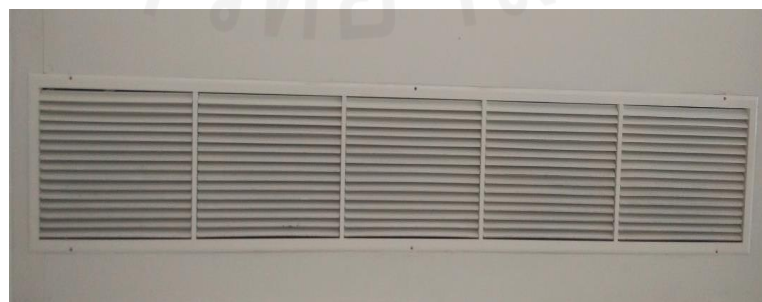
Fig. 3.9. Extract grilles mounted on ceiling
