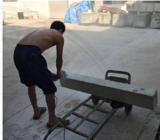
(b) Clean the surface of RC beams to remove dust and dirt.
