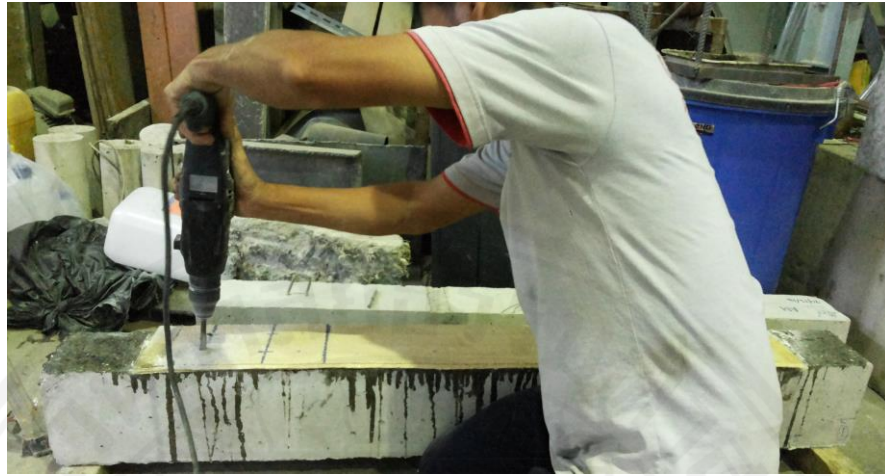
(a) The anchor holes were drilled at desired locations
