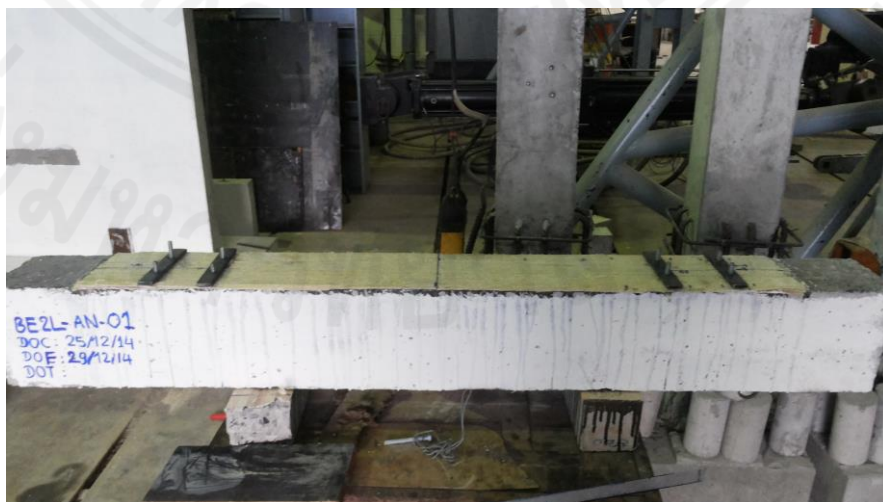
(c) After sika was fully hardened (24 hours), steel plates were placed and nuts were tightened.
