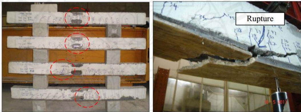
Figure 2.7 Failure modes of tested RC beams
