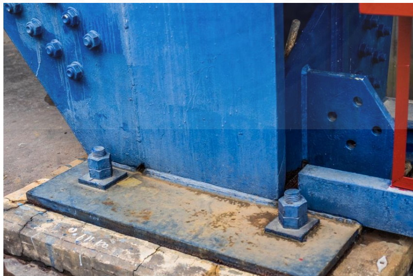
Fig 4.37 The intensity change of anti-corrosive paint in Power Plant D
