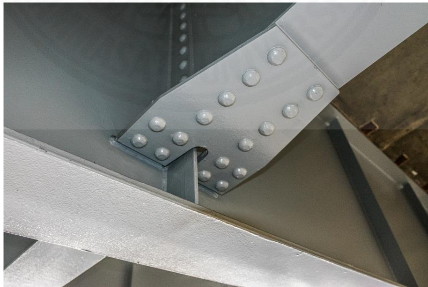
Fig 4.55 Bolt connection of steel girder at Highway Bridge B
