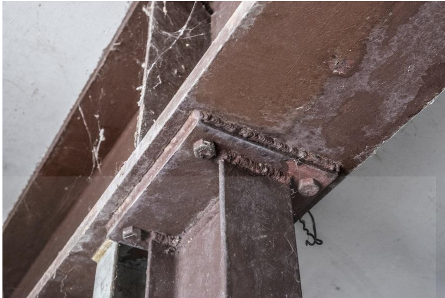
Fig 4.47 Weld connection of the steel structure in Power Plant E
