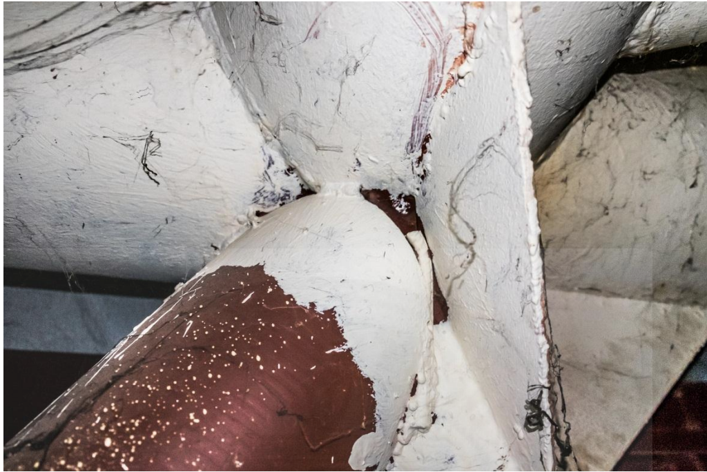
Fig 4.89 Discontinuity of weld on Roof Structure B (1)
