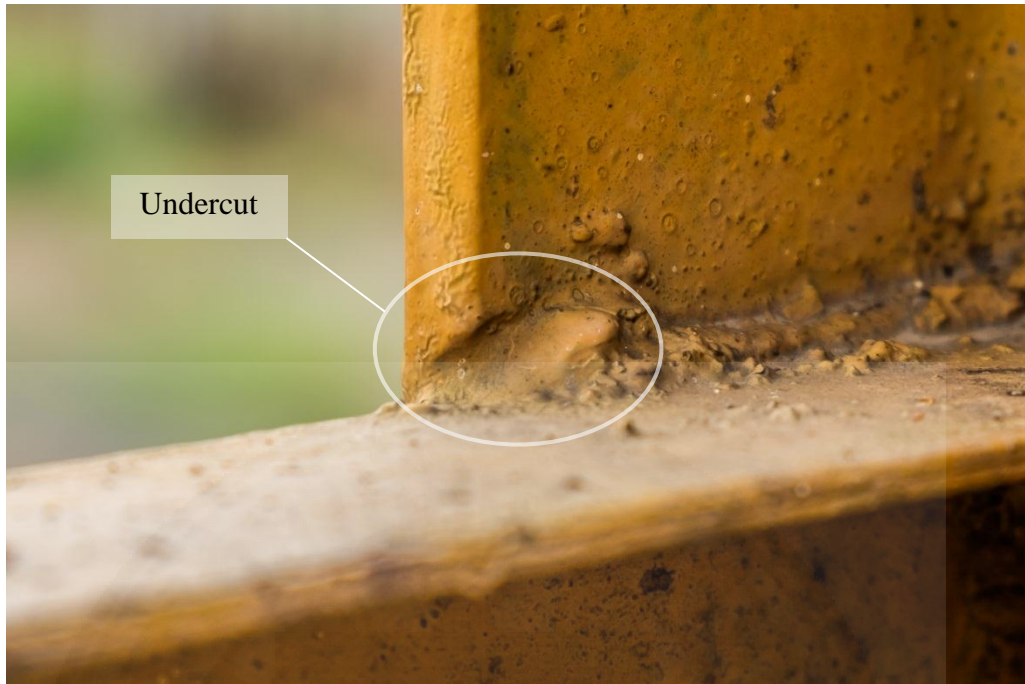
Fig 4.70 Welding defects on Billboard A (joint 4)
