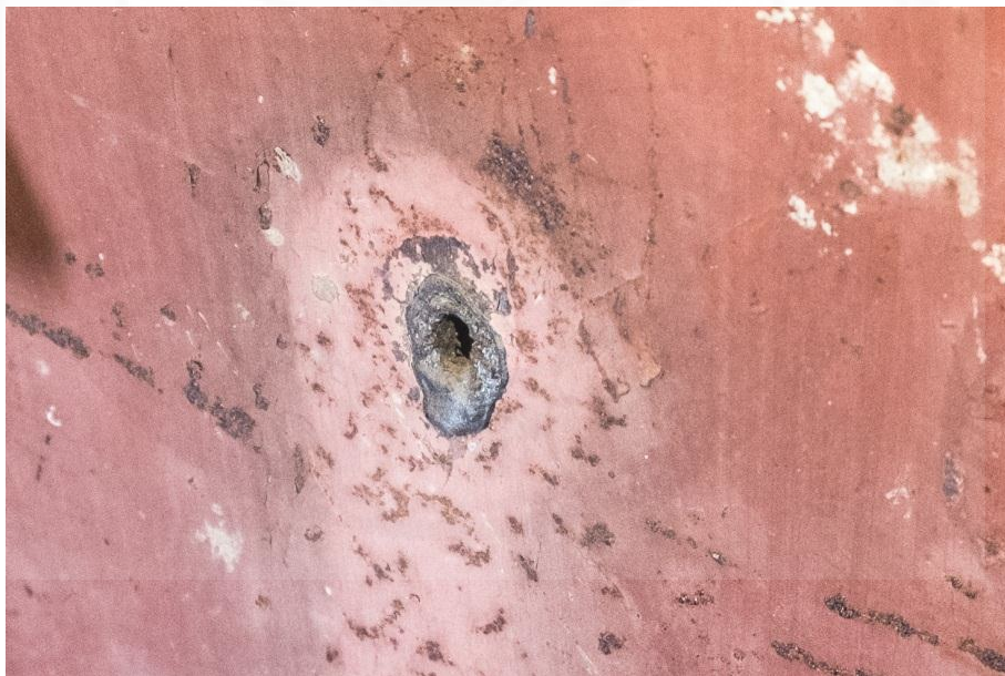
Fig 4.81 Damage from welding process on the steel column (2)
