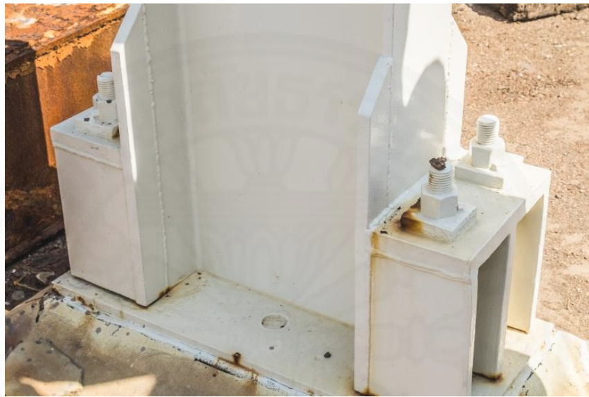
Fig 4.21 Weld and bolt connection of steel column at Power Plant B
