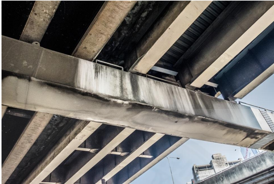
Fig 4.51 Lichen on the steel surface at Highway Bridge A
