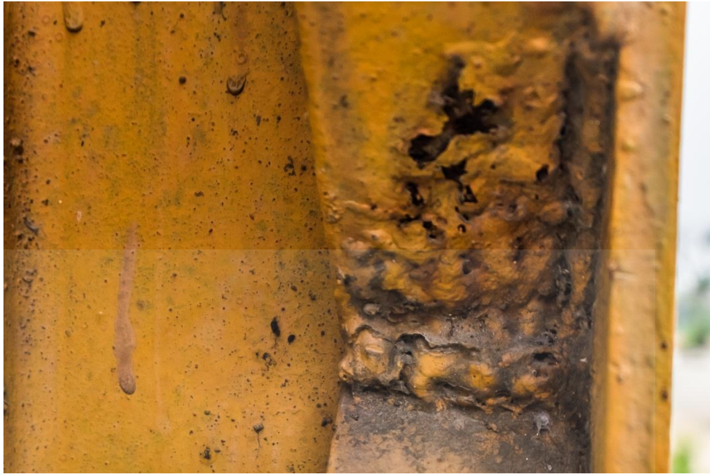
Fig 4.60 Blistering and rusting of paint on Billboard A (3)
