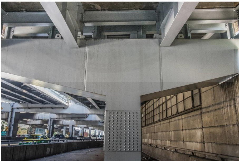
Fig 4.52 Painted steel surface of Highway Bridge B (1)
