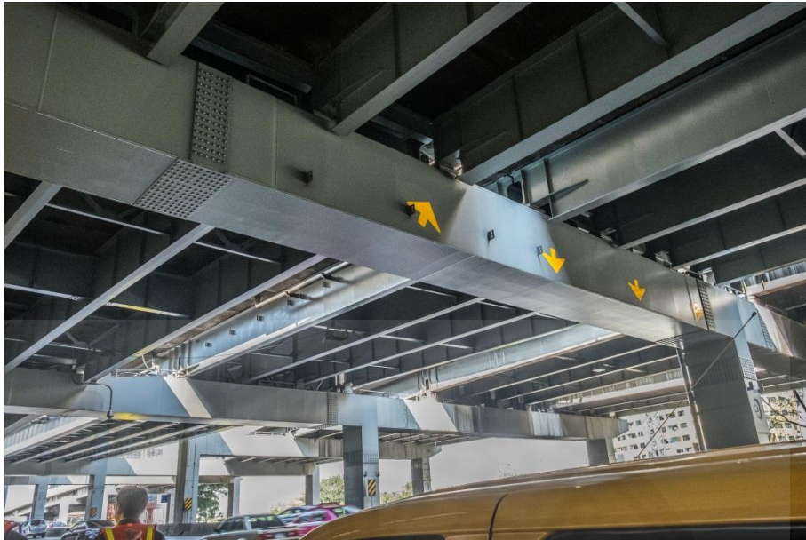
Fig 4.49 Overview of Highway Bridge B
