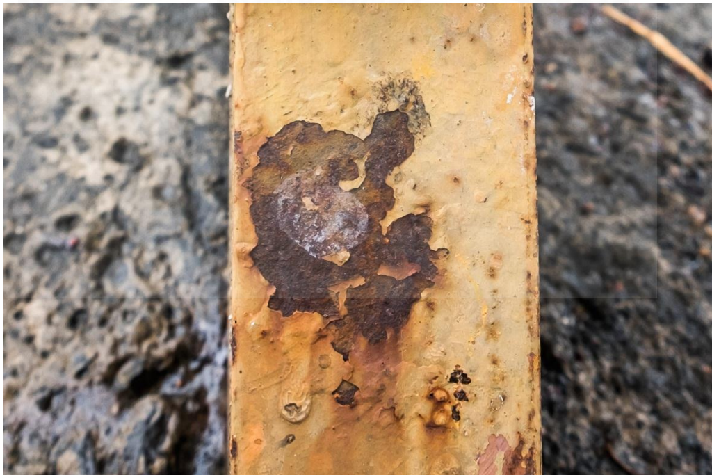
Fig 4.61 Flaking and rusting of paint on Billboard A (1)
