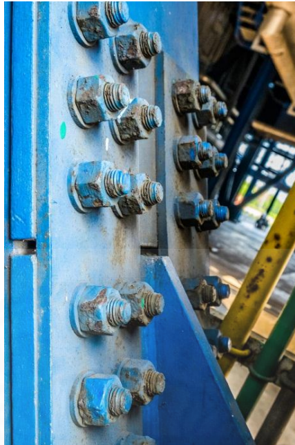
Fig 4.9 Blistering and flaking of paint on bolt at Power Plant A (2)
