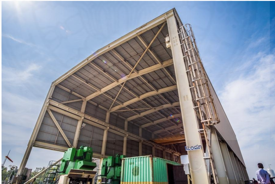
Fig 4.11 Steel Structure in Power Plant B (1)
