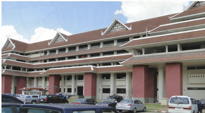
Fig 4.73 Overview of the Roof Structure A
