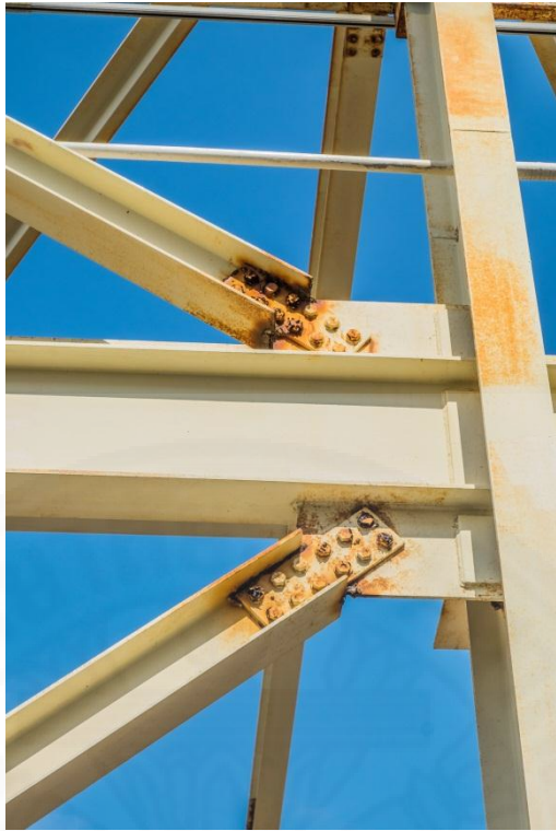
Fig 4.14 Corrosion on the steel bolt connection at Power Plant B (1)
