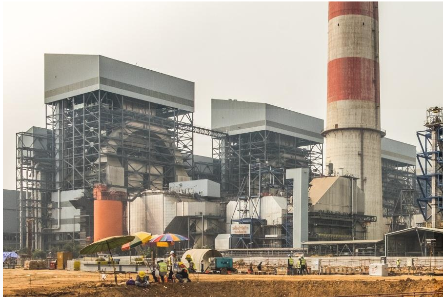
Fig 4.23 Steel structure in Power Plant C (1)
