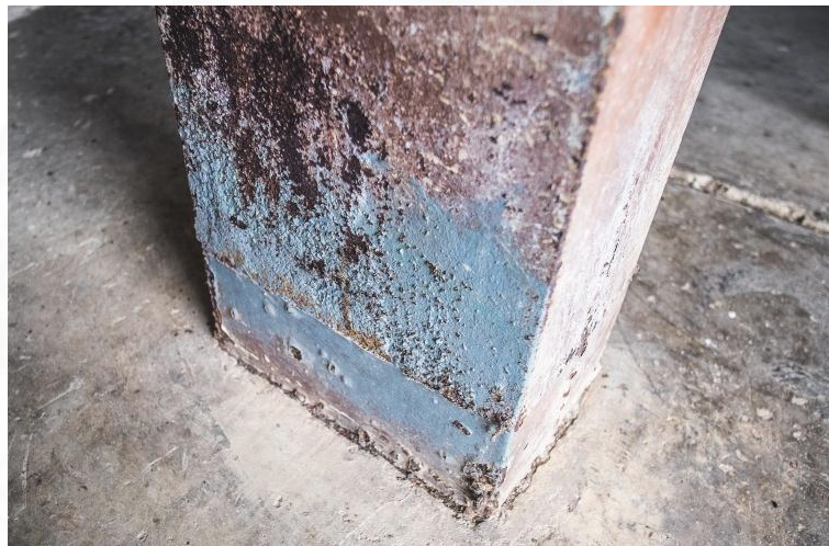
Fig 4.41 Corrosion on the steel column in Power Plant E
