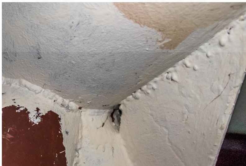
Fig 4.88 Small Porosity on the weld connection at Roof Structure B
