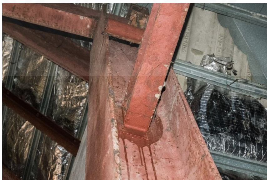
Fig 4.83 Weld connection of beam-column at Roof Structure A
