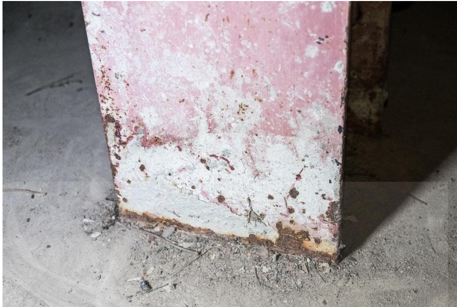
Fig 4.76 Corrosion on the steel column at Roof Structure A (3)
