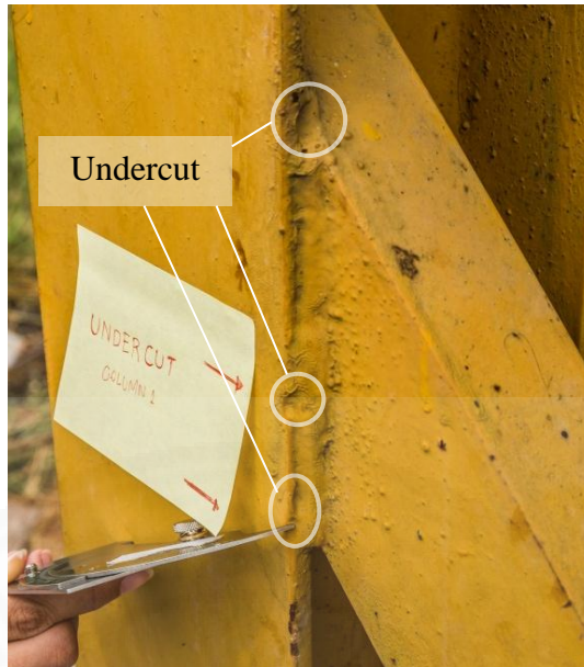
Fig 4.68 Welding defects on Billboard A (joint 2)
