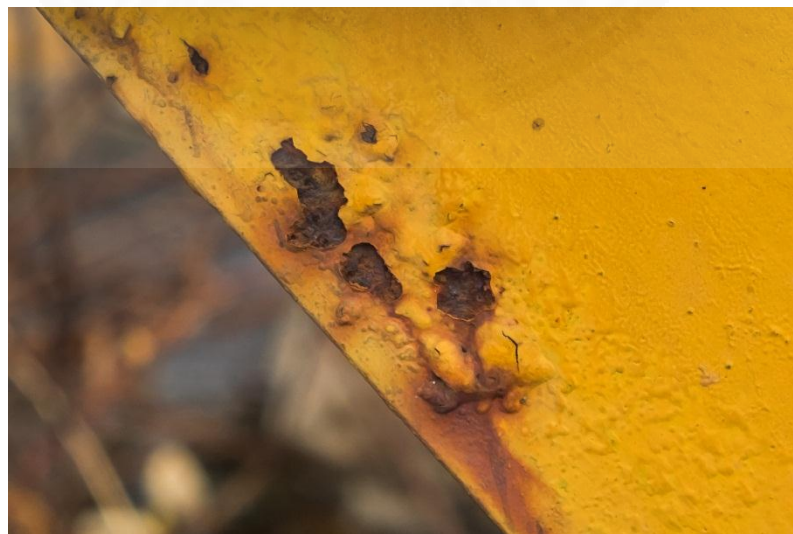
Fig 4.59 Blistering and rusting of paint on Billboard A (2)
