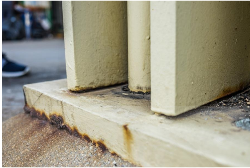
Fig 4.20 Space between steel column and steel plate in Power Plant B
