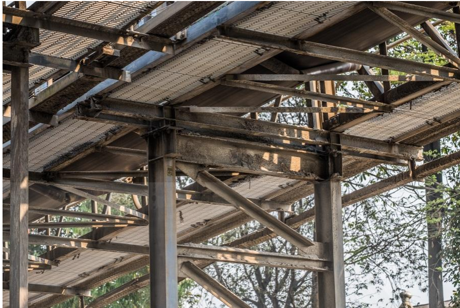
Fig 4.28 Deterioration on the steel conveyor at Power Plant C (1)
