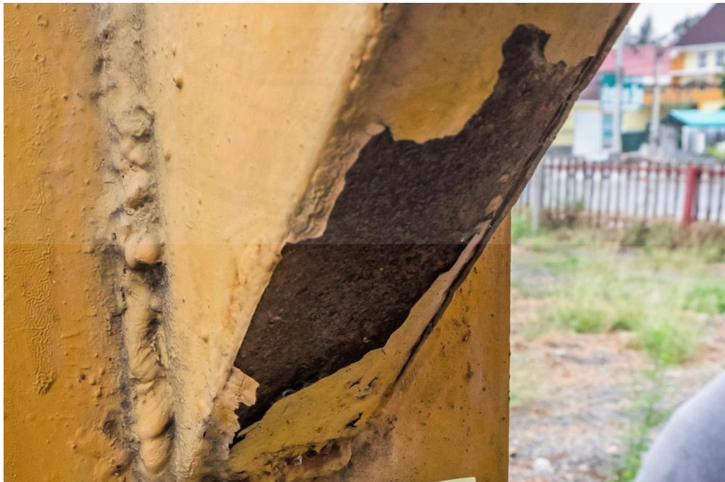
Fig 4.63 Flaking and rusting of paint on Billboard A (3)
