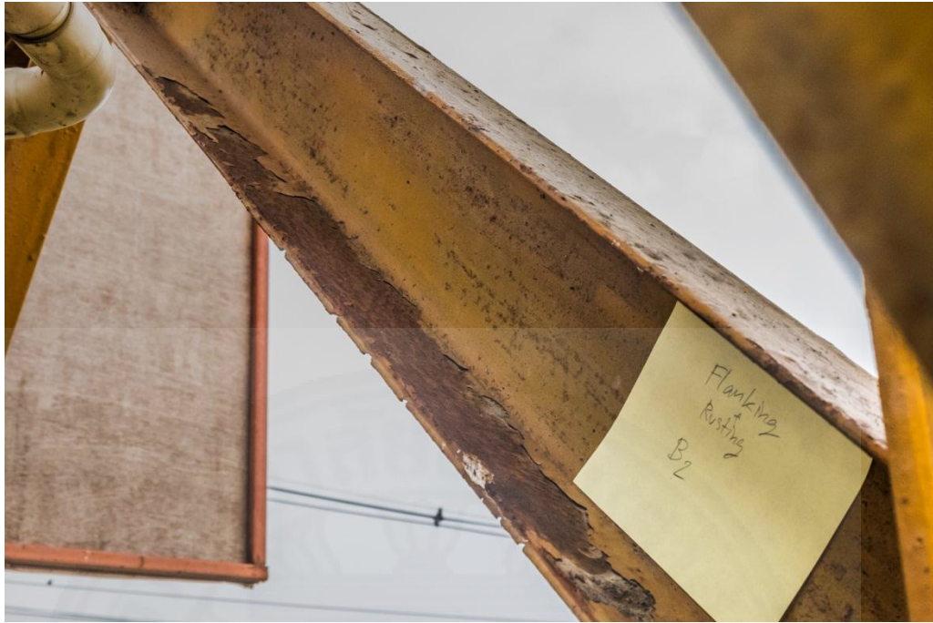
Fig 4.62 Flaking and rusting of paint on Billboard A (2)
