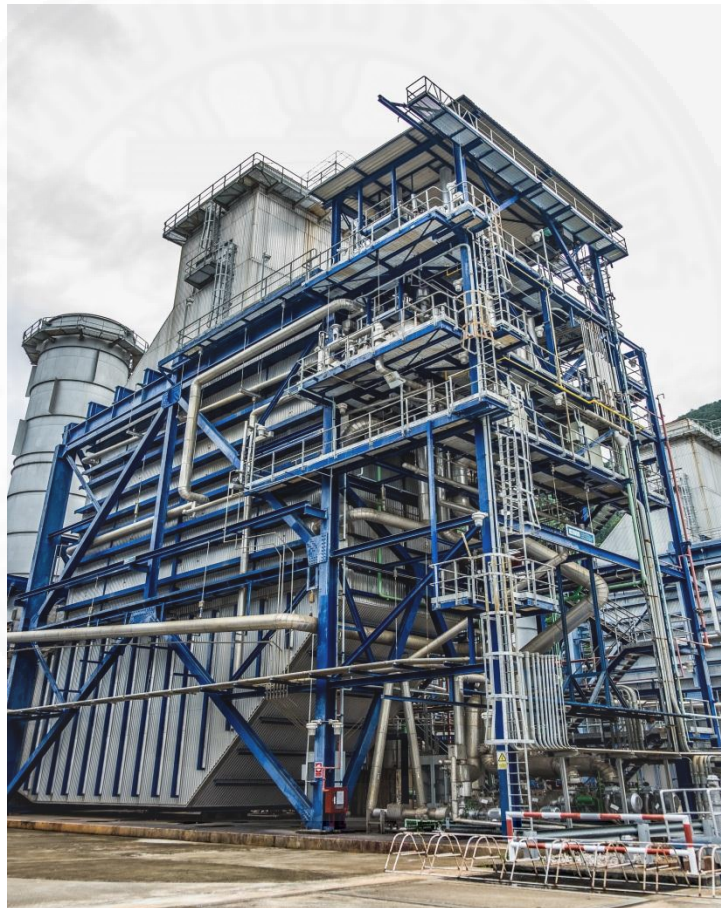
Fig 4.34 Steel Structure in Power Plant D
