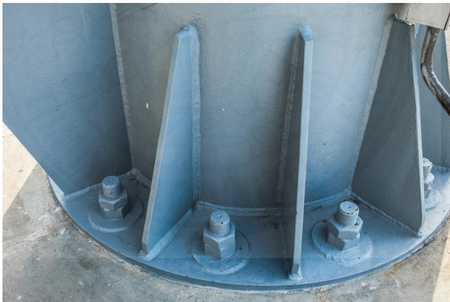
Fig 4.10 Weld and bolt connection of steel column at Power Plant A
