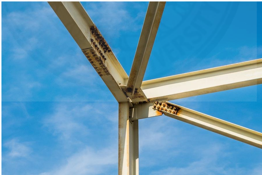
Fig 4.15 Corrosion on the steel bolt connection at Power Plant B (2)
