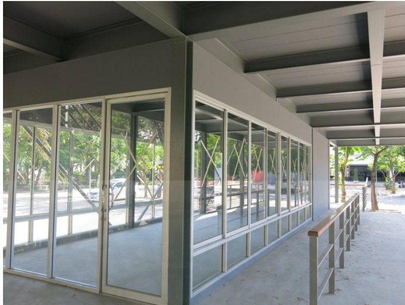
Fig 4.93 Overview of a steel coating as Steel Structure A
