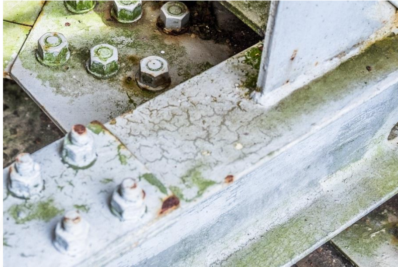
Fig 4.43 Cracking of the anti-corrosive paint in Power Plant E
