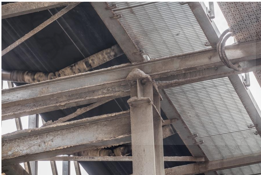
Fig 4.29 Deterioration on the steel conveyor at Power Plant C (2)
