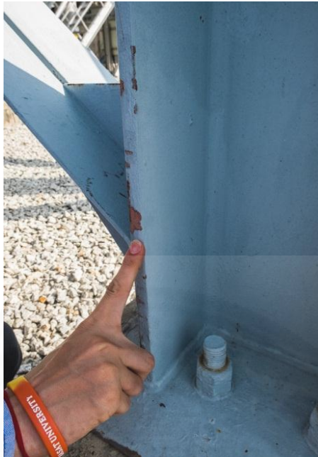
Fig 4.5 Flaking of anti-corrosive paint at Power Plant A
