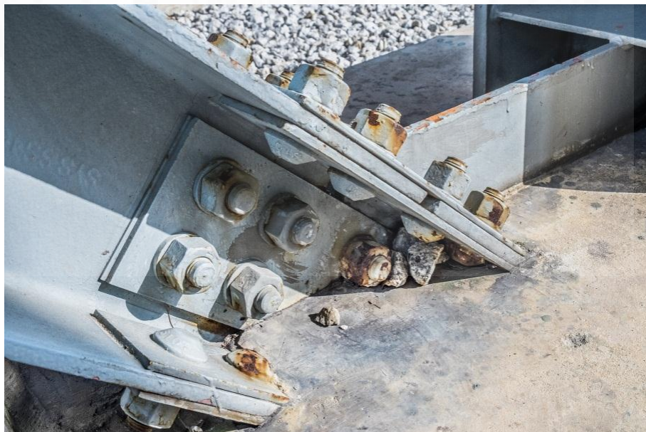
Fig 4.8 Blistering and flaking of paint on bolt at Power Plant A (1)
