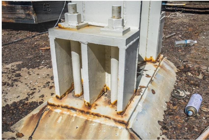
Fig 4.16 Corrosion on the steel column connection at Power Plant B
