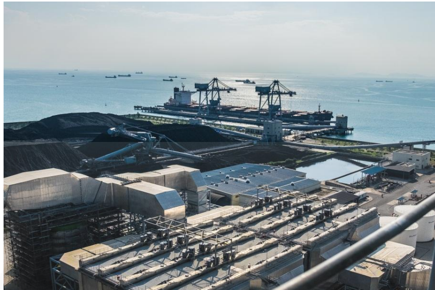
Fig 4.1 Overview of Power Plant A (1)
