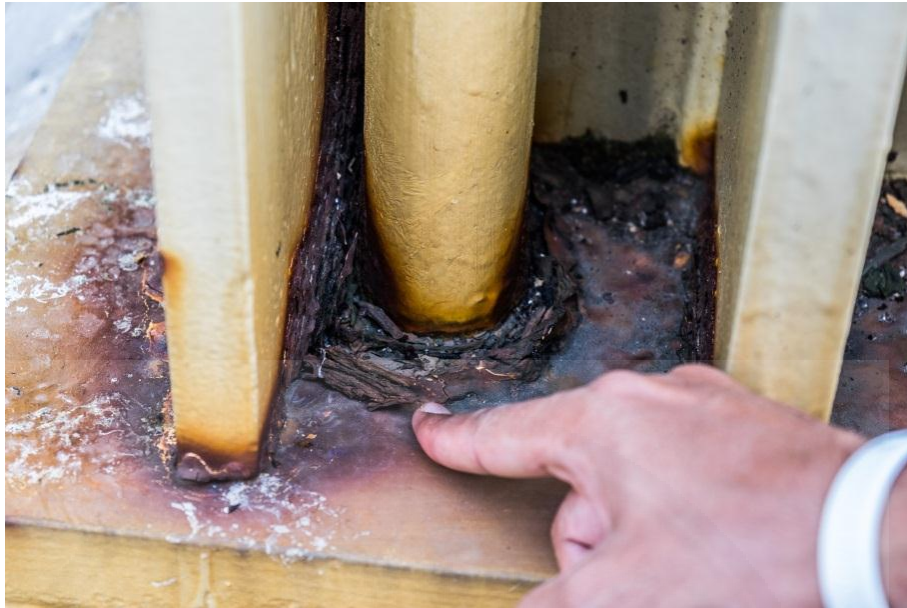
Fig 4.18 Corrosion at the bottom of the column in Power Plant B (1)
