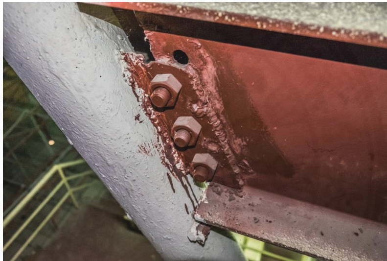
Fig 4.87 Undercut on the steel weld connection as Roof Structure B
