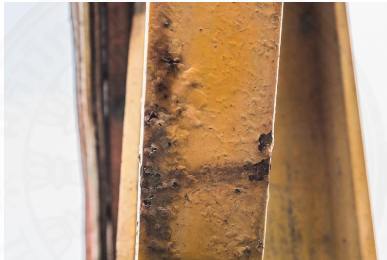
Fig 4.58 Blistering and rusting of paint on Billboard A (1)
