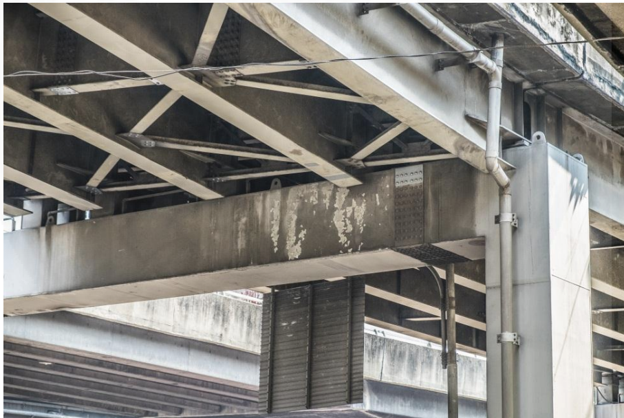
Fig 4.50 Flaking of paint on steel surface at Highway Bridge A
