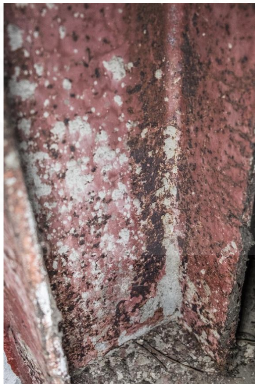
Fig 4.77 Corrosion on the steel column at Roof Structure A (4)
