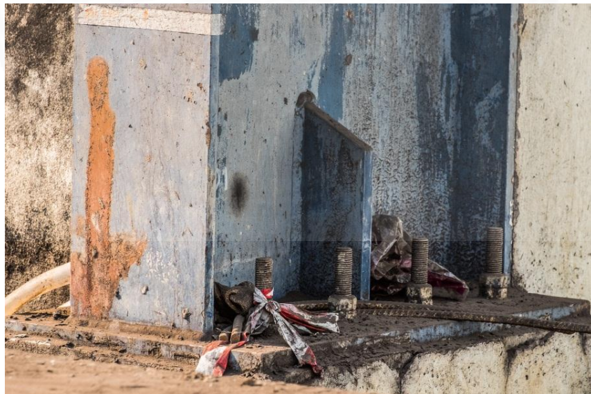
Fig 4.33 Steel weld and bolt connection at Power Plant C
