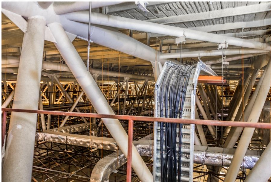
Fig 4.85 Overview of Roof Structure B (2)
