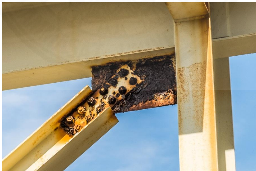
Fig 4.13 Severe corrosion on steel bolt connection in Power Plant B
