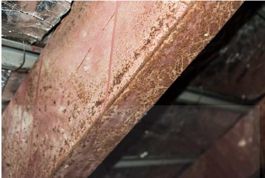
Fig 4.78 Corrosion on the steel beam at Roof Structure A
