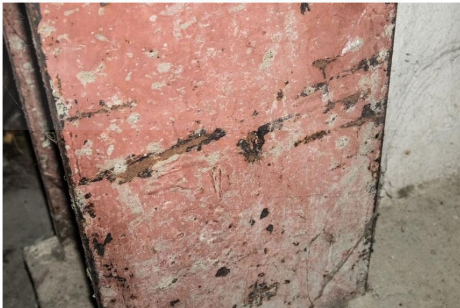
Fig 4.75 Corrosion on the steel column at Roof Structure A (2)
