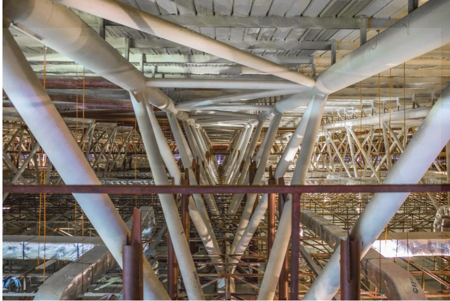
Fig 4.84 Overview of Roof Structure B (1)
