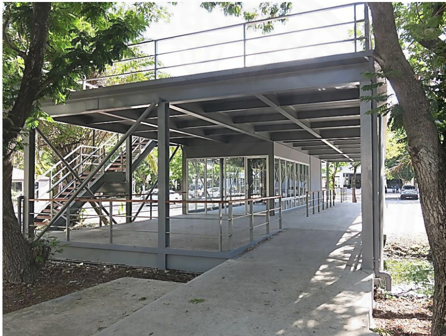
Fig 4.92 Overview of Steel Structure A
