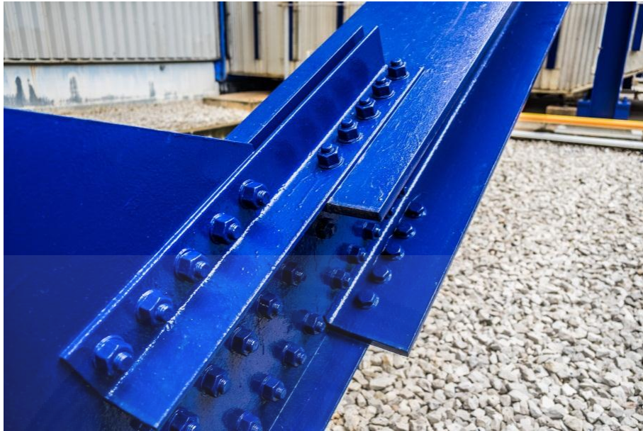
Fig 4.39 Steel bolted connection at Power Plant D
