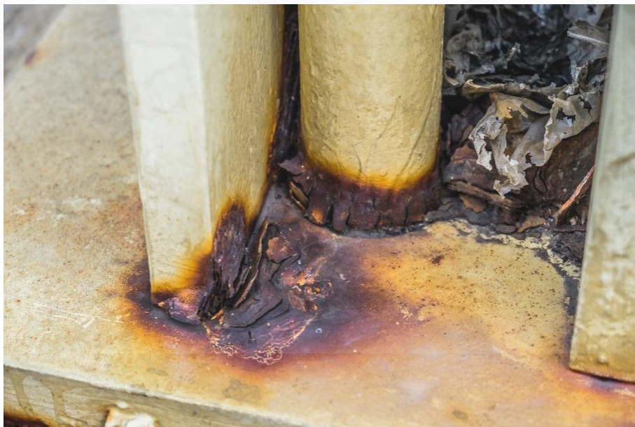
Fig 4.19 Corrosion at the bottom of the column in Power Plant B (2)
