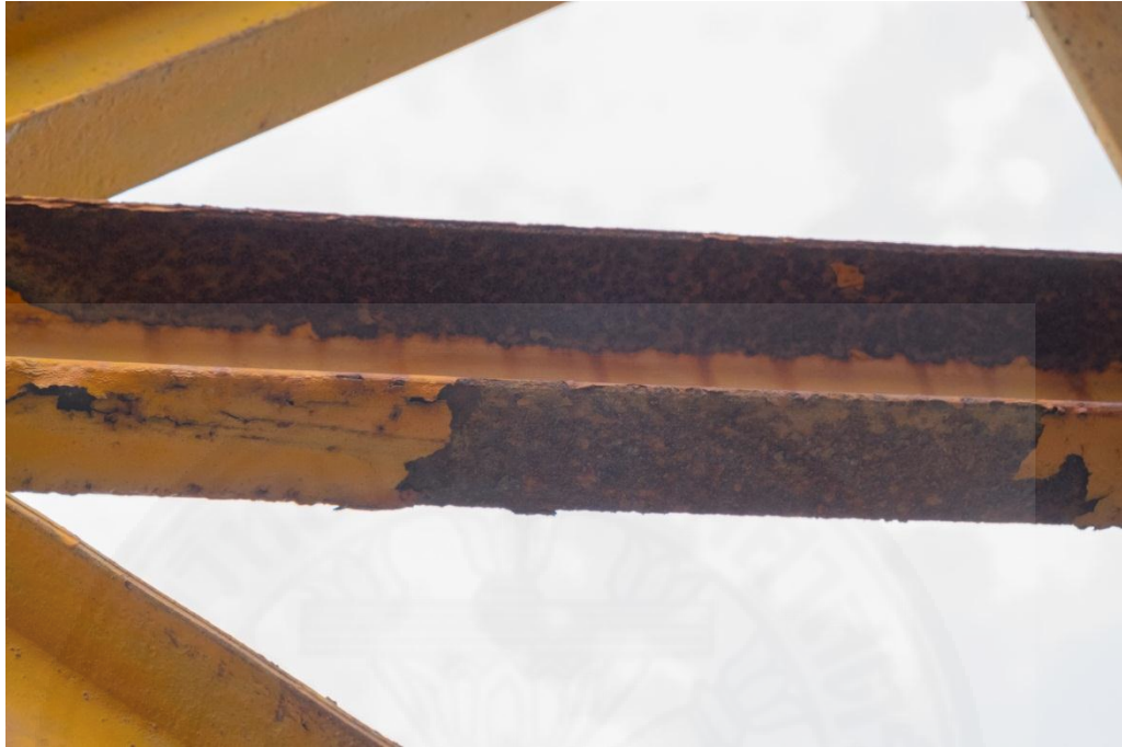
Fig 4.64 Flaking and rusting of paint on Billboard A (4)
