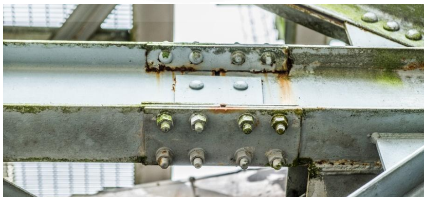
Fig 4.42 Rusting and blistering on the steel bolt in Power Plant E
