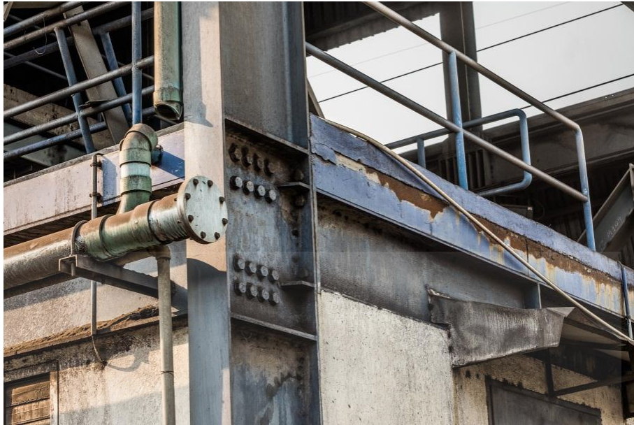
Fig 4.27 Flaking and corrosion of the steel coating at Power Plant C
