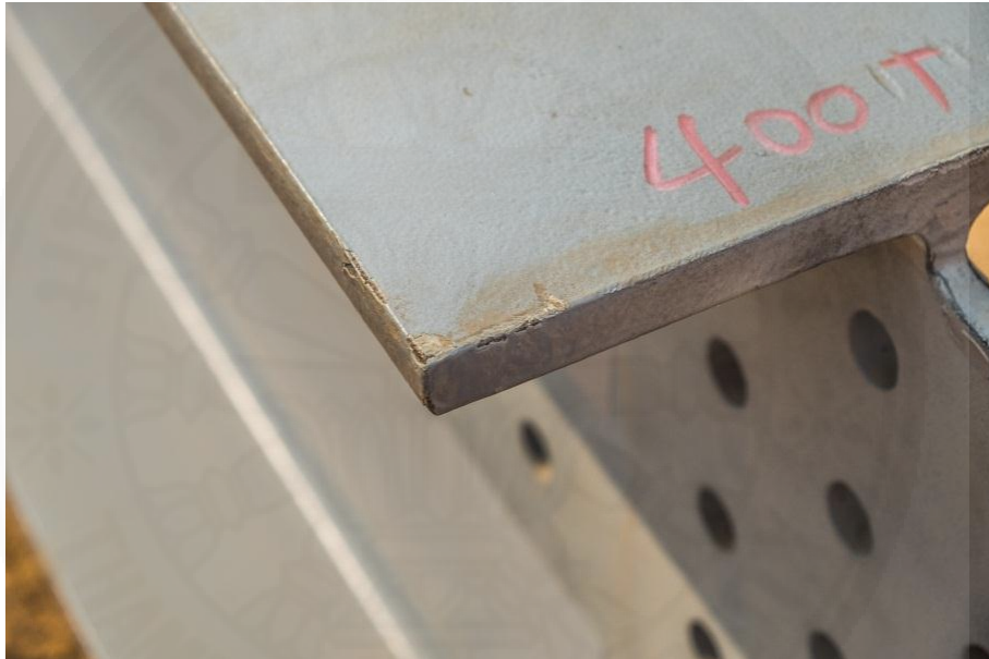
Fig 4.26 Anti-corrosive coating on the steel section at Power Plant C
