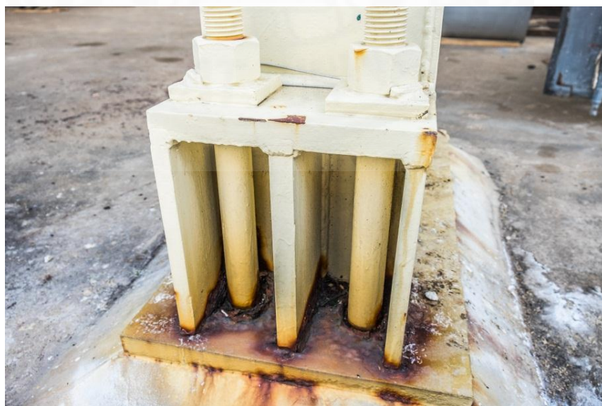
Fig 4.17 Corrosion on the steel column connection at Power Plant B
