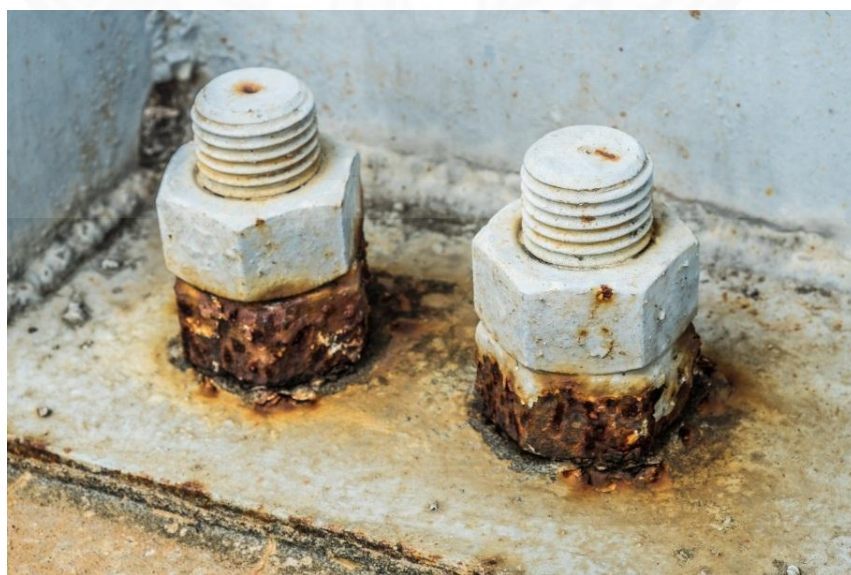
Fig 4.44 Corrosion damage on the bolt connection at Power Plant E
