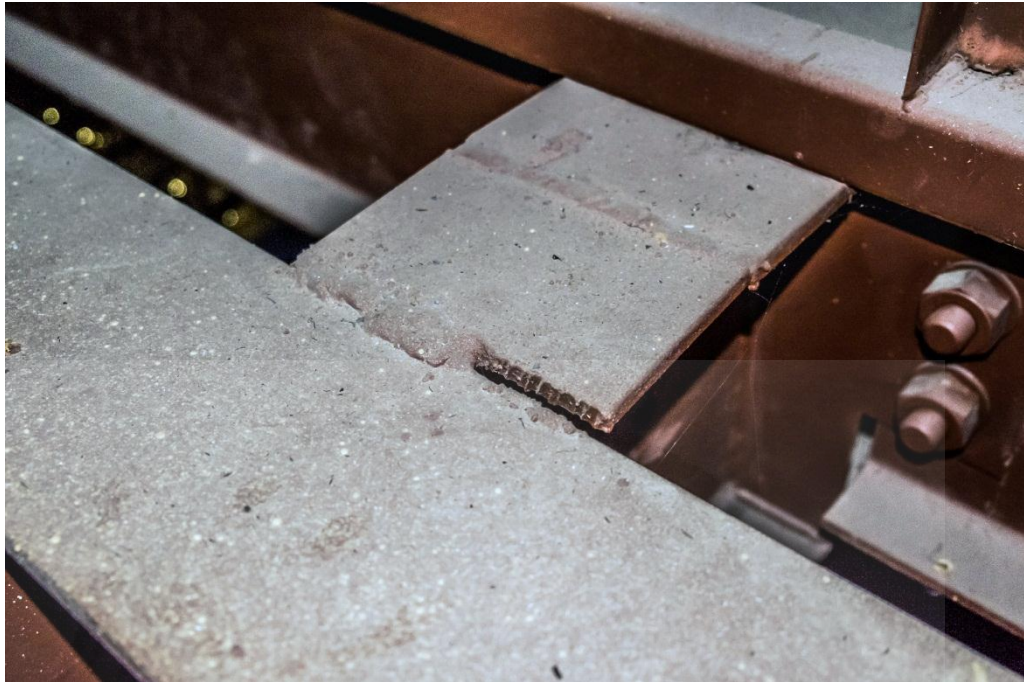
Fig 4.91 Missing weld on the beam girder at Roof Structure B
