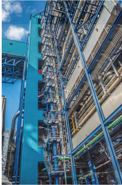
Fig 4.3 Steel structure in Power Plant A (2)
