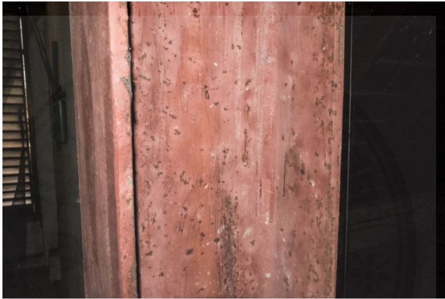
Fig 4.74 Corrosion on the steel column at Roof Structure A (1)
