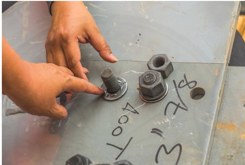
Fig 4.30 Indicator washer used in bolt connection at Power Plant C
