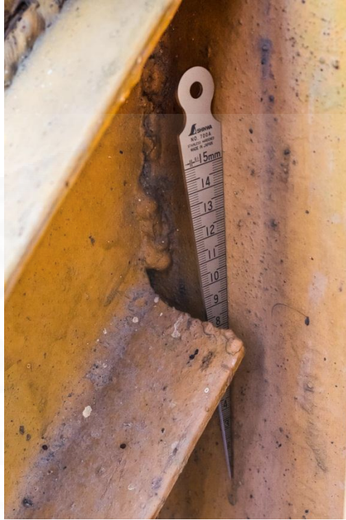
Fig 4.72 Welding defects on Billboard A (joint 6)
