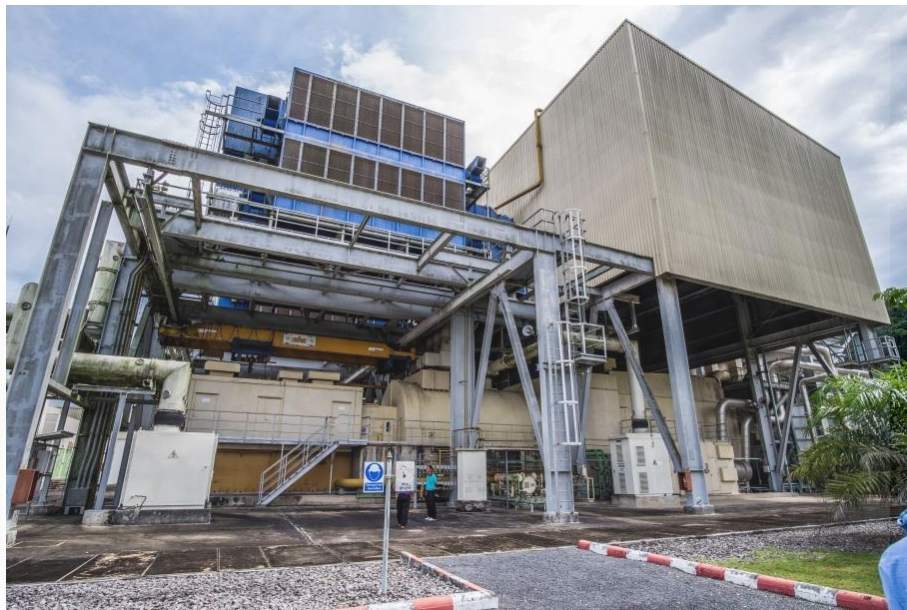
Fig 4.40 Overview of the steel structure in Power Plant E
