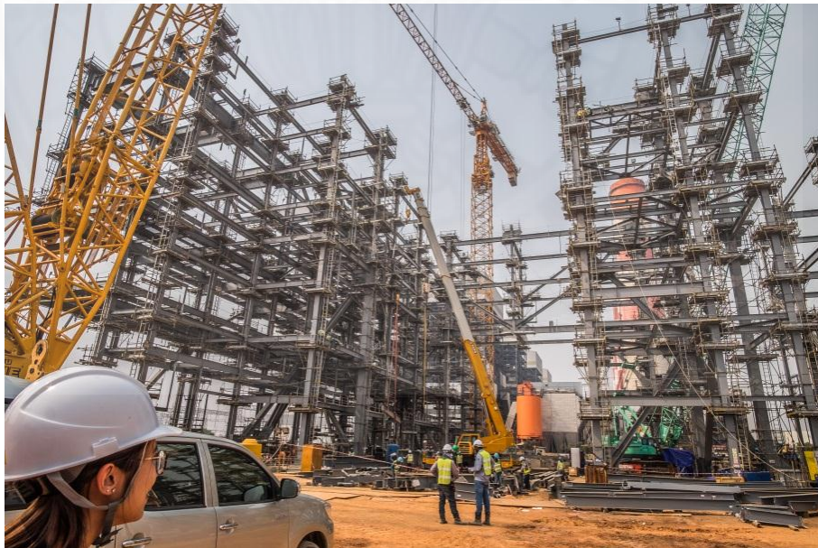
Fig 4.22 Construction site of Power Plant C
