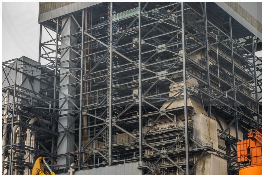
Fig 4.24 Steel structure in Power Plant C (2)
