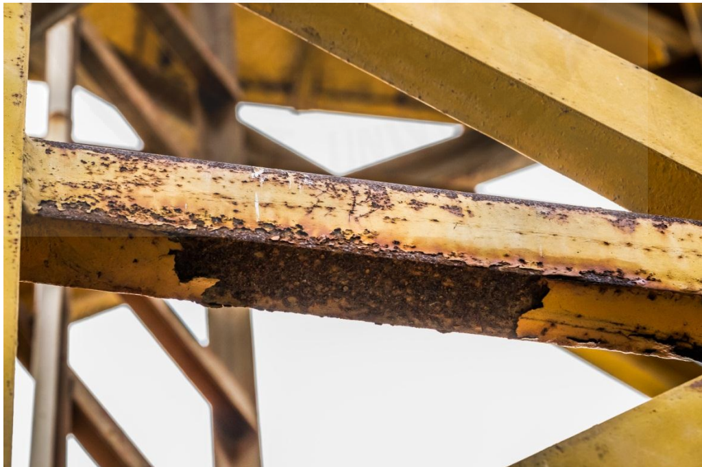
Fig 4.65 Flaking and rusting of paint on Billboard A (5)
