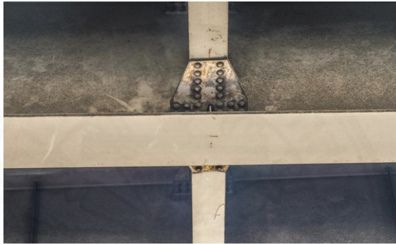
Fig 4.54 Bolt connection of steel girder at Highway Bridge A
