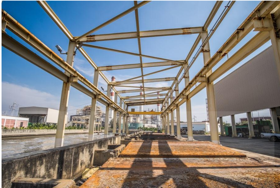
Fig 4.12 Steel Structure in Power Plant B (2)
