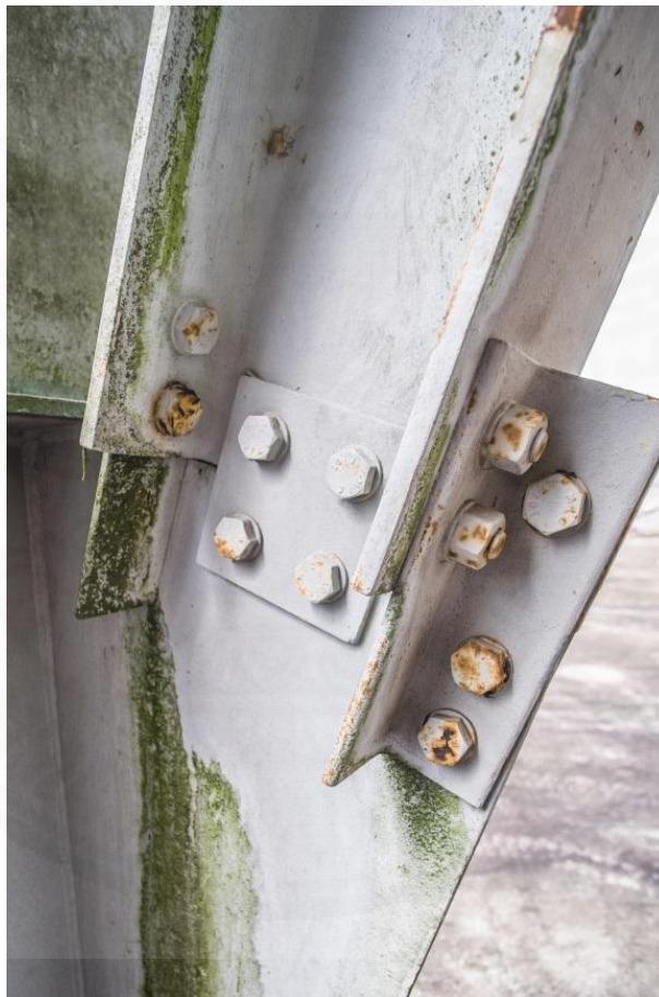
Fig 4.46 Bolt connection of the steel structure in Power Plant E
