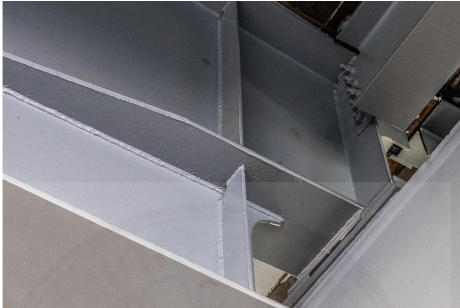
Fig 4.56 Weld connection of the steel section at Highway Bridge B
