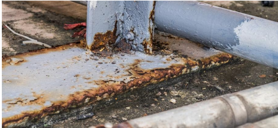
Fig 4.45 Flaking of the anti-corrosive paint as Power Plant E
