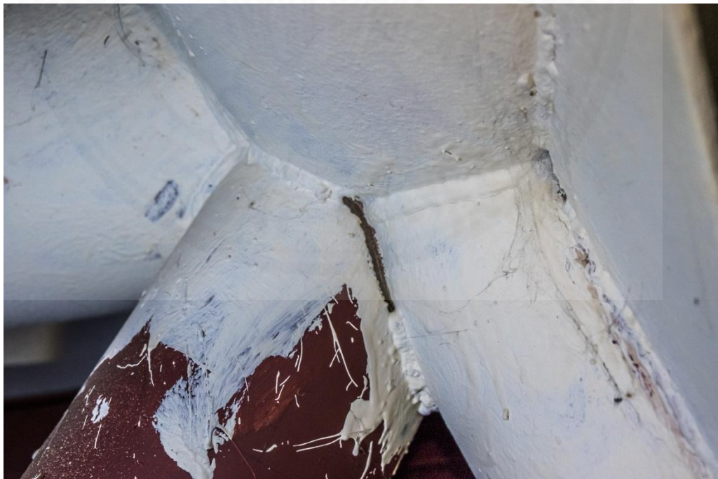
Fig 4.90 Discontinuity of weld on Roof Structure B (2)
