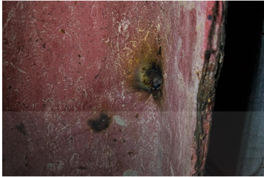
Fig 4.82 Damage from welding process on the steel column (3)
