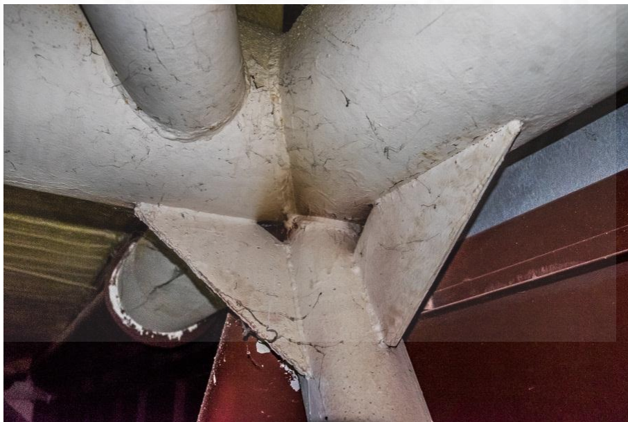
Fig 4.86 Intensity change of steel coating at Roof Structure B
