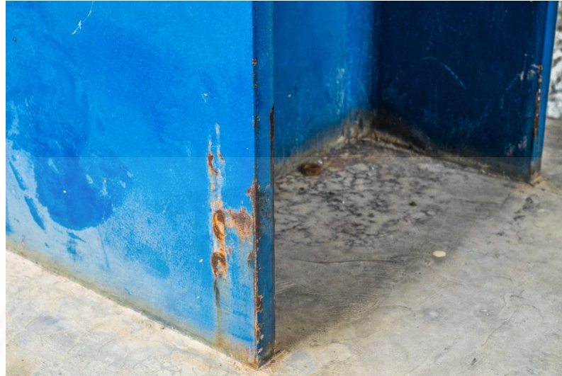
Fig 4.7 Rusting of anti-corrosive paint at Power Plant A
