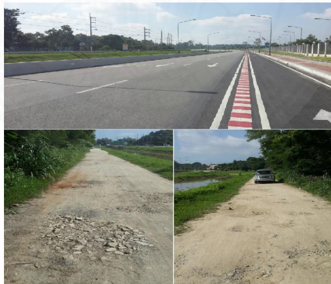
Fig. 4.1 Road condition characteristic good road(top) and bad road(under)
