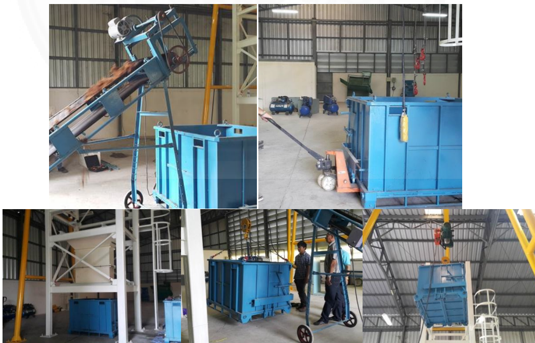
Figure 4.19 Primary checks of reactor and STR equipment
