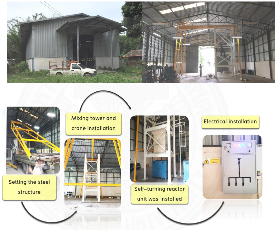
Figure 3.21 Plant modification and setting up the equipment
