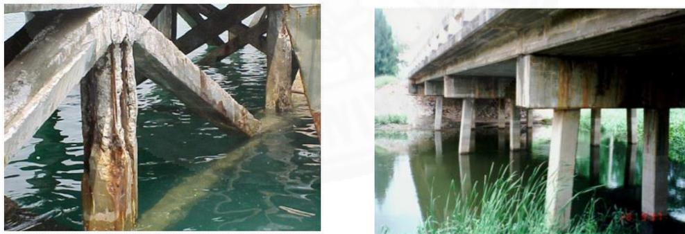
Fig. 2.5 Steel corrosion caused by the chloride
