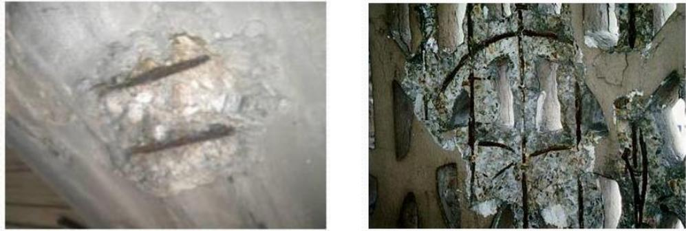
Fig 2.3 Steel corrosion caused by the ingress of carbonation
