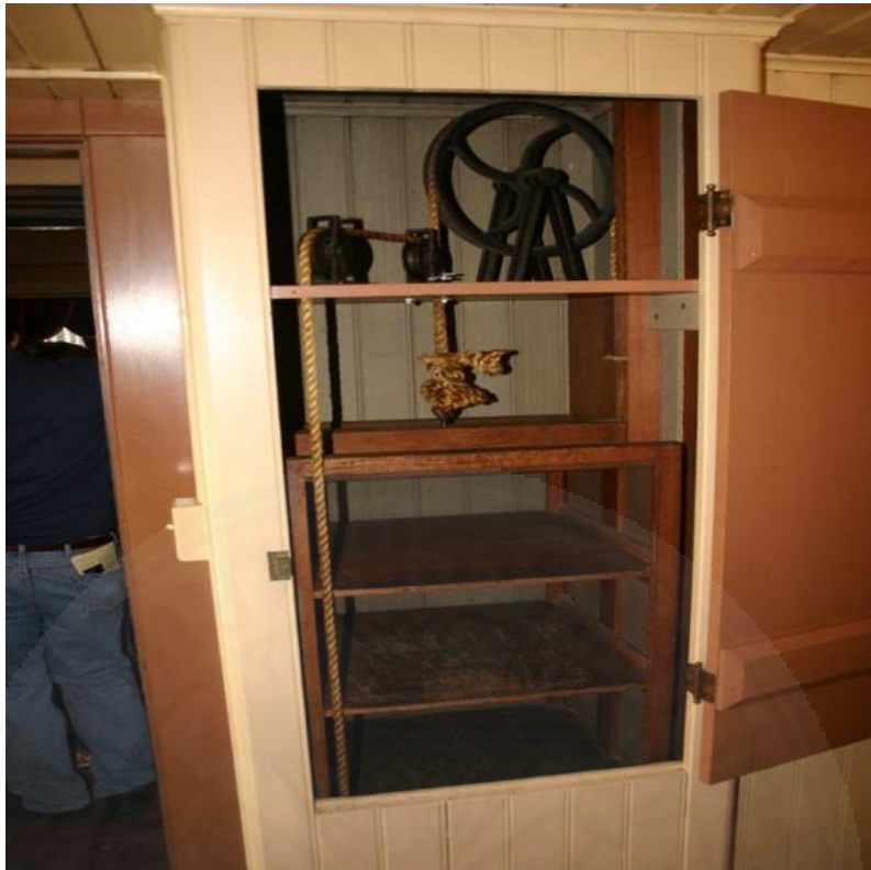
Figure 2.7 Manual Dumbwaiter Source : Herbie T. Mann
