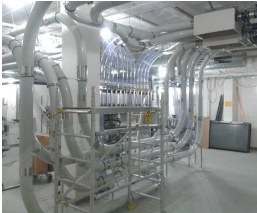
Figure 2.1 Interchange Station Source : Swisslog
