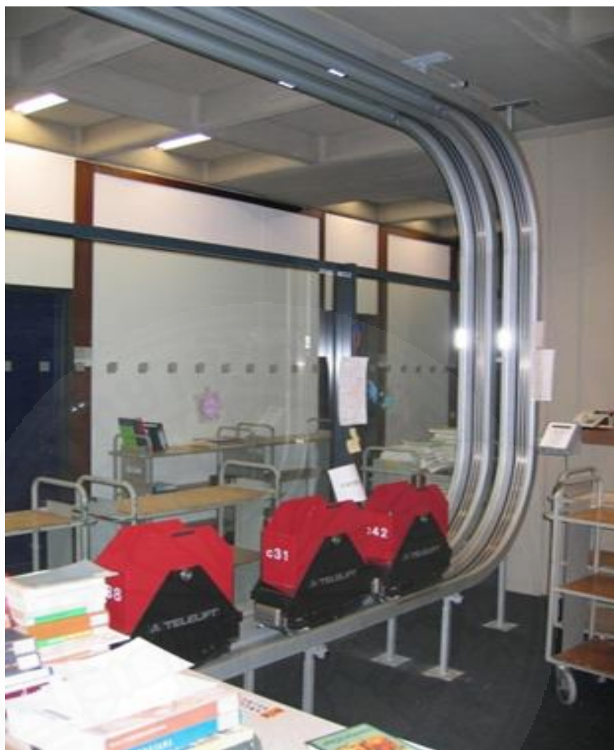
Figure 2.14 Telelift used in library Source : Telelift GmbH.
