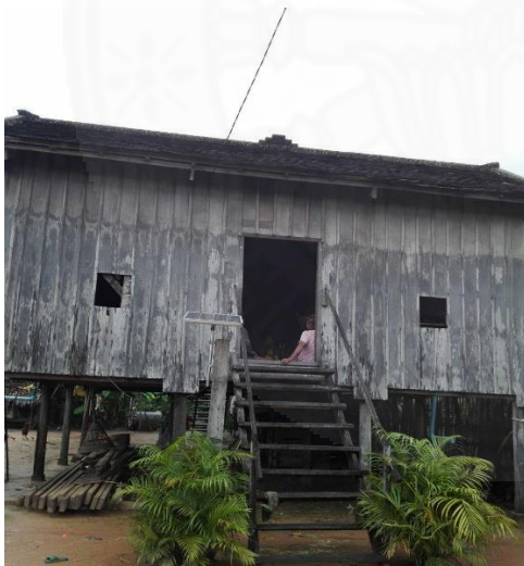
Wooden house with SHS
