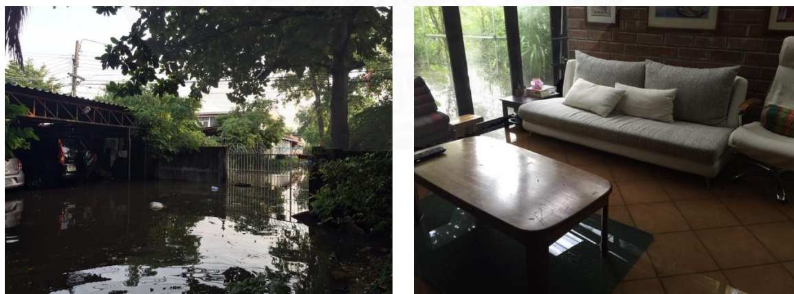
Figure 4.11 Condition inside the house after heavy rainfall for 2-3 hours, causing it to be impossible to access in and out the community.
