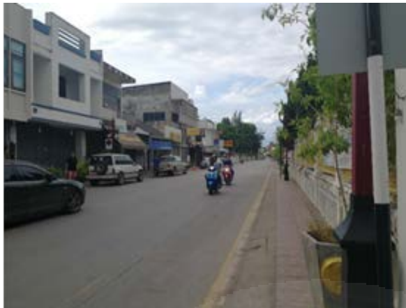
Figure 6.10 Existing footpath condition on Chaing Mai - Lamphun road.
