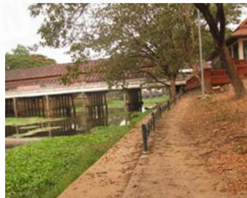
Figure 4.40 Riverfront walkway. Source: Researcher, 18 October 2018.
