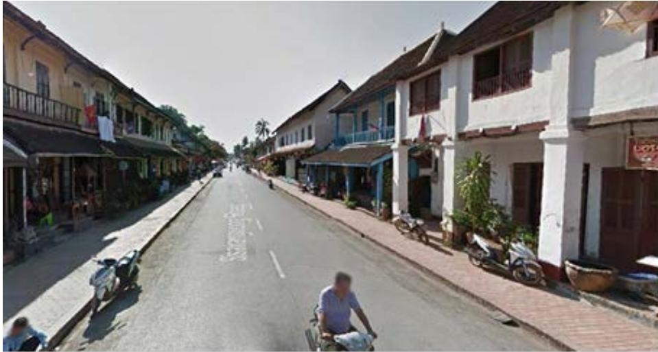
Figure 2.36 Underground electric wires/utilities for a clear and beautiful scenic view in Laung Prabang town, Laos. Retrieved October 22, 2018.
