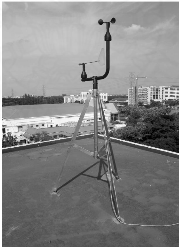
Figure 4.1 Installation of three-cup type anemometer and wind vane on building rooftop.
