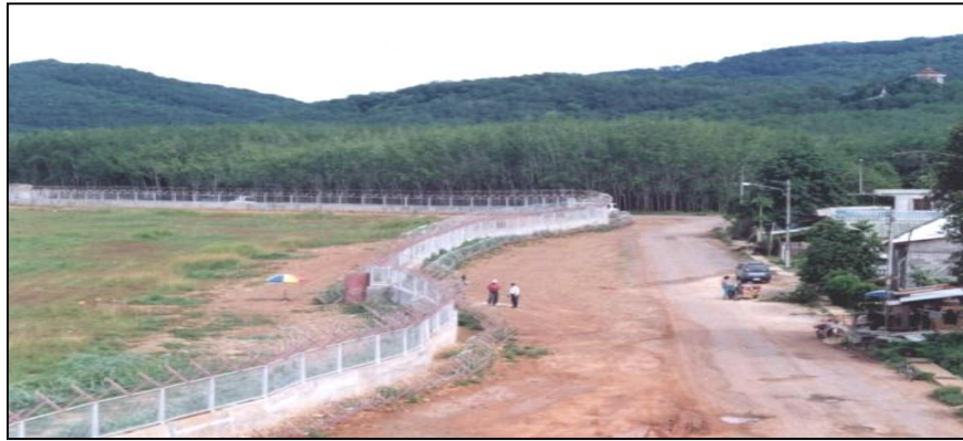
Figure 3.4: The single barrier at Padang Besar Songkhla Province/Perlis State Source: Land Boundaries Committee (LBC) Thailand – Malaysia)
