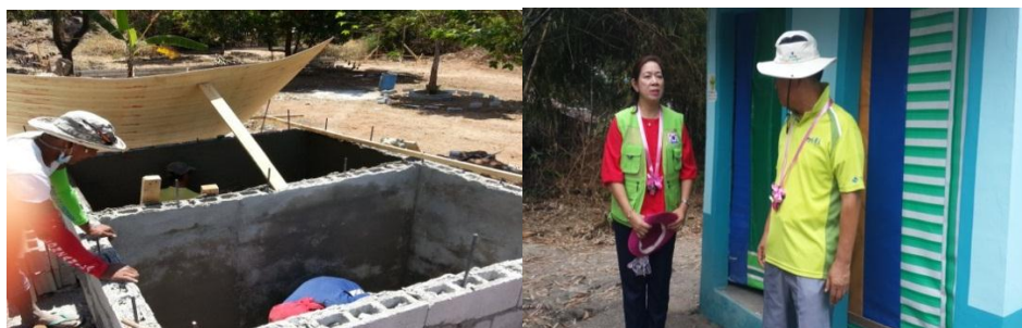
Installation of public toilet
