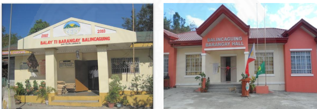
Construction of community hall (before and after)
