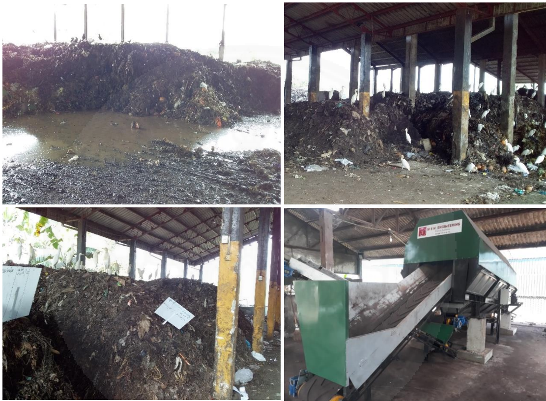
Figure 3.3 Key components of the composting plant.
