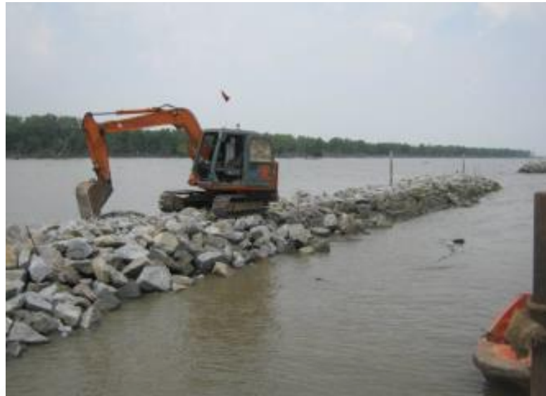
Figure 1.1 Rock embankment construction. (Ashimori industries Co., Ltd.)
