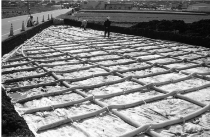
Figure 2.17 Application of LFR system for road construction [Okamoto, M (2009)]
