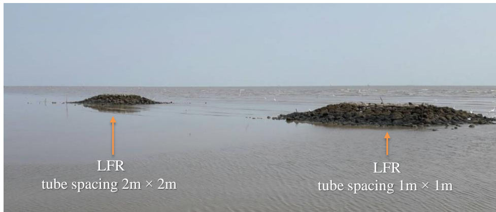
Figure 3.9 Embankments with LFR systems being monitored
