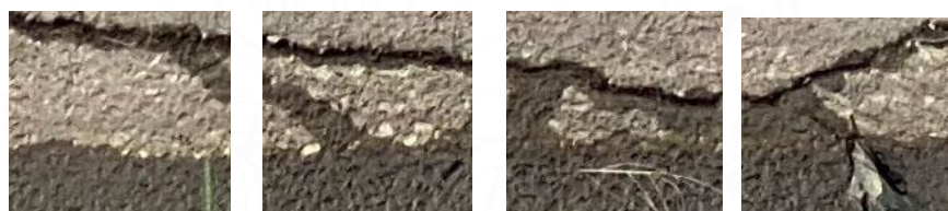
Crack Patch
