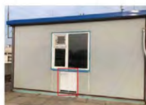
Figure 3: A ventilator installed below the window of a test room (the southern view).
